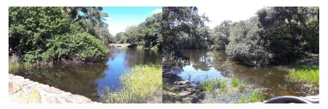
26) Bridge at #4 north green-repair leaning wall and hole forming along cartpath. The wall behind the rip-rap is leaning, leaving a void between the two walls. Rainfall can get between the wall and rip-rap causing erosion. The hole along the edge of the cartpath is weakening the structural integrity of the path. \$42,000.00
