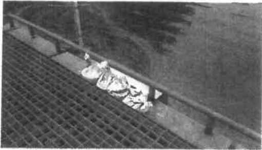
Nursery Rd-sandbags blocking weir to raise water level. Removed.
