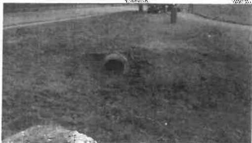
Between 10 and 11N on East Lake Woodlands Parkway-clear mouth of culvert. $ 1,145.00
