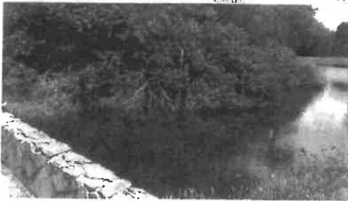
15 th south tee from bridge Remove low hanging tree limbs $ 2,590.00 for both pictures
