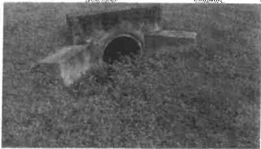
Sun Trust at Woodlands Drive-clear mouth of culvert $ 730.00
