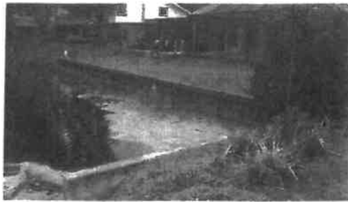
Beneath Pine Lake Dr in Woodlands Estates-check water flow with dye test $ 100.00
